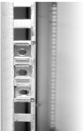
FIGURE 1-22. Cage nuts for a fixed mount
